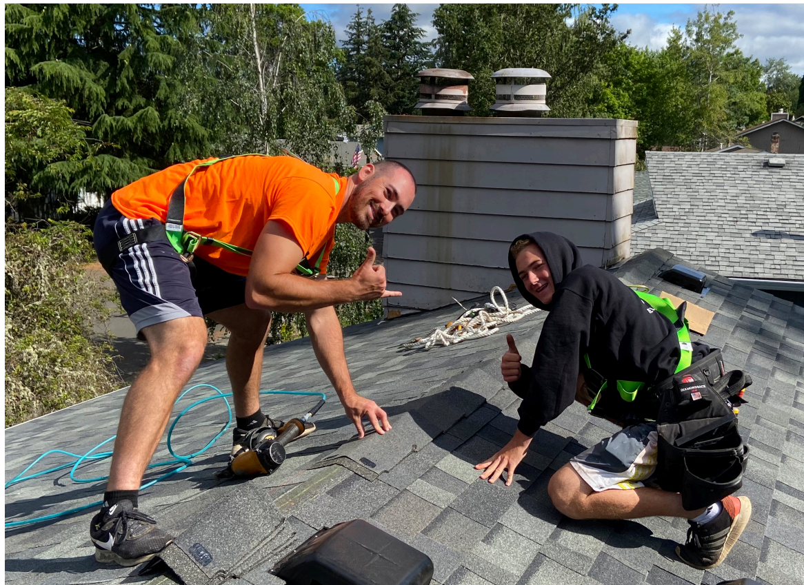
Carson Puppo (right) and his older brother Aaron (left) pose for a photo during a roofing job. The two brothers are the co-founders of Peak Performance roofing. Photo provided by Carson Puppo.
